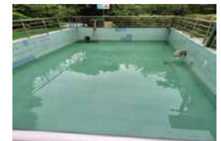
改進污水處理工藝 improving wastewater treatment processes
