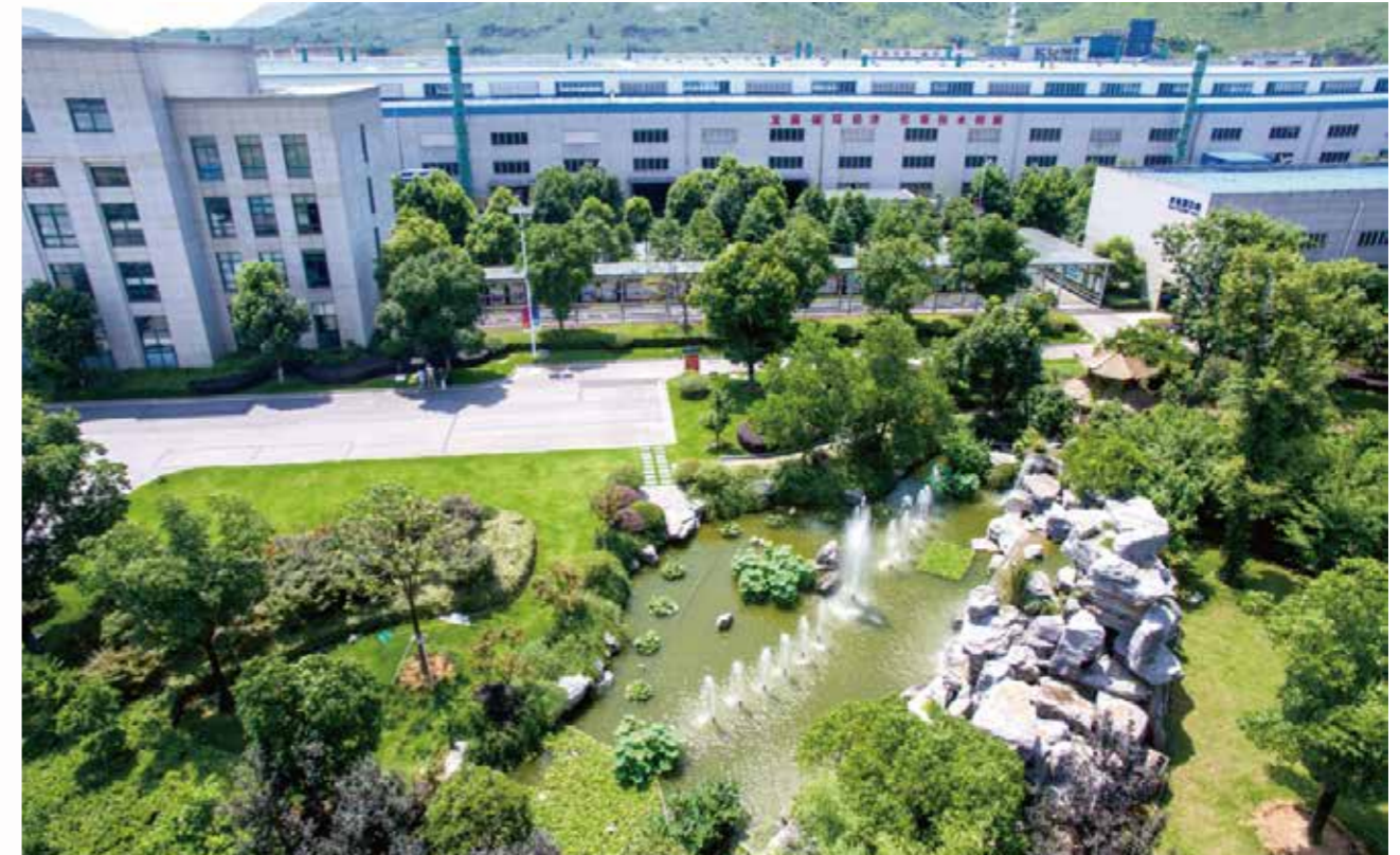
鉛蓄電池循環基地 Lead Battery Recycling Base
