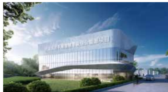
嘉興平湖儲能項目 Energy Storage Project in Pinghu, Jiaxing City
